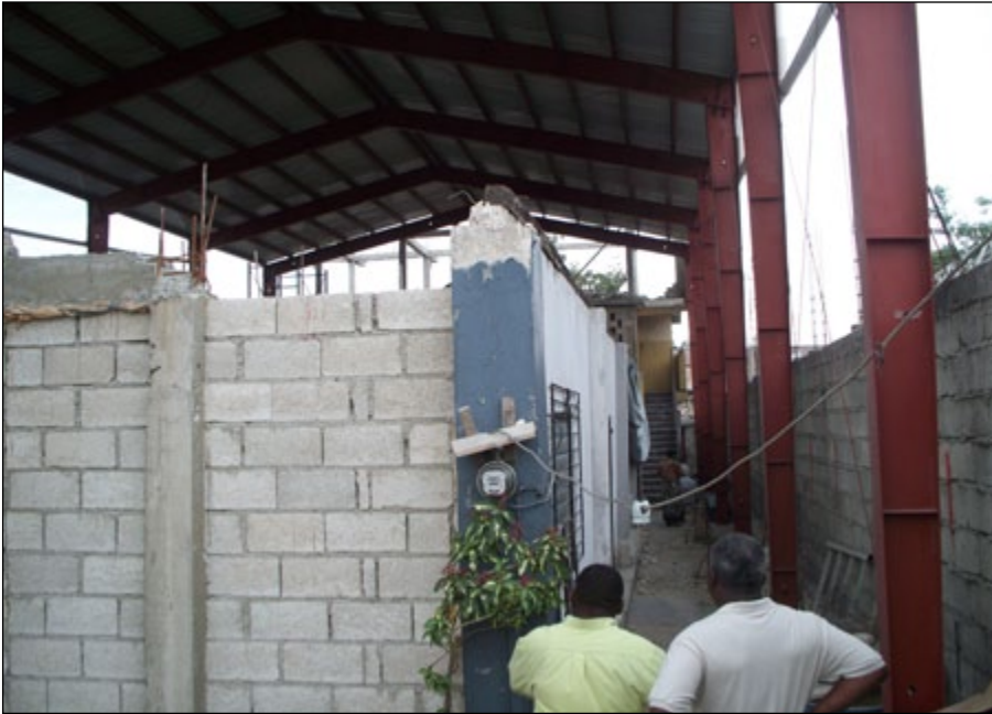
A church within a church. Spacious and raised steel structure allows for balcony to the rear and sides of building.
